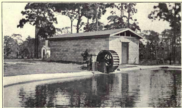
Fig. 2.—Artesian well used for power belonging to H. T. Bowden, Melbourne, Brevard County. The water from the artesian well affords power by which water is pumped from a nearby shallow well.
